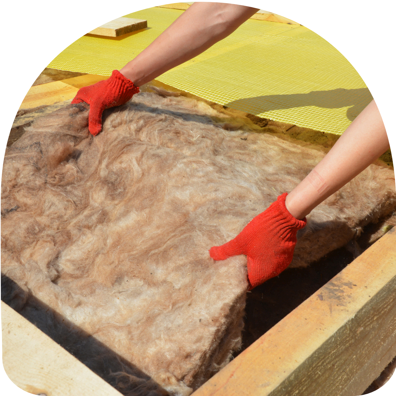
Insulation installation. Credit: Canva stock image
