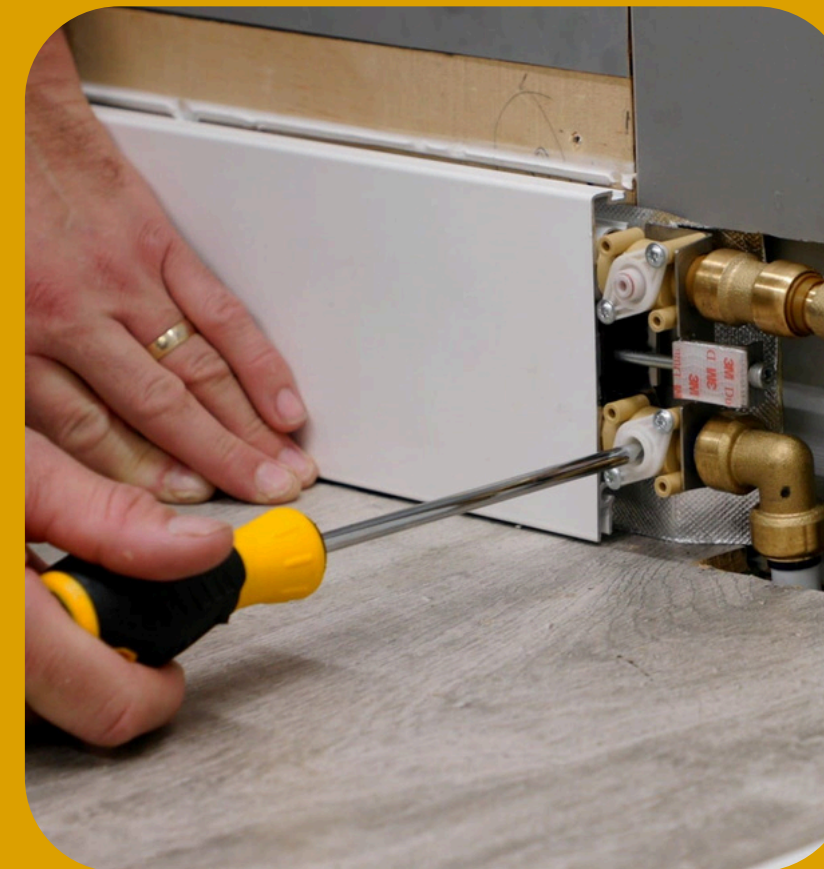
ThermaSkirt installation. Credit: Discrete Heat
