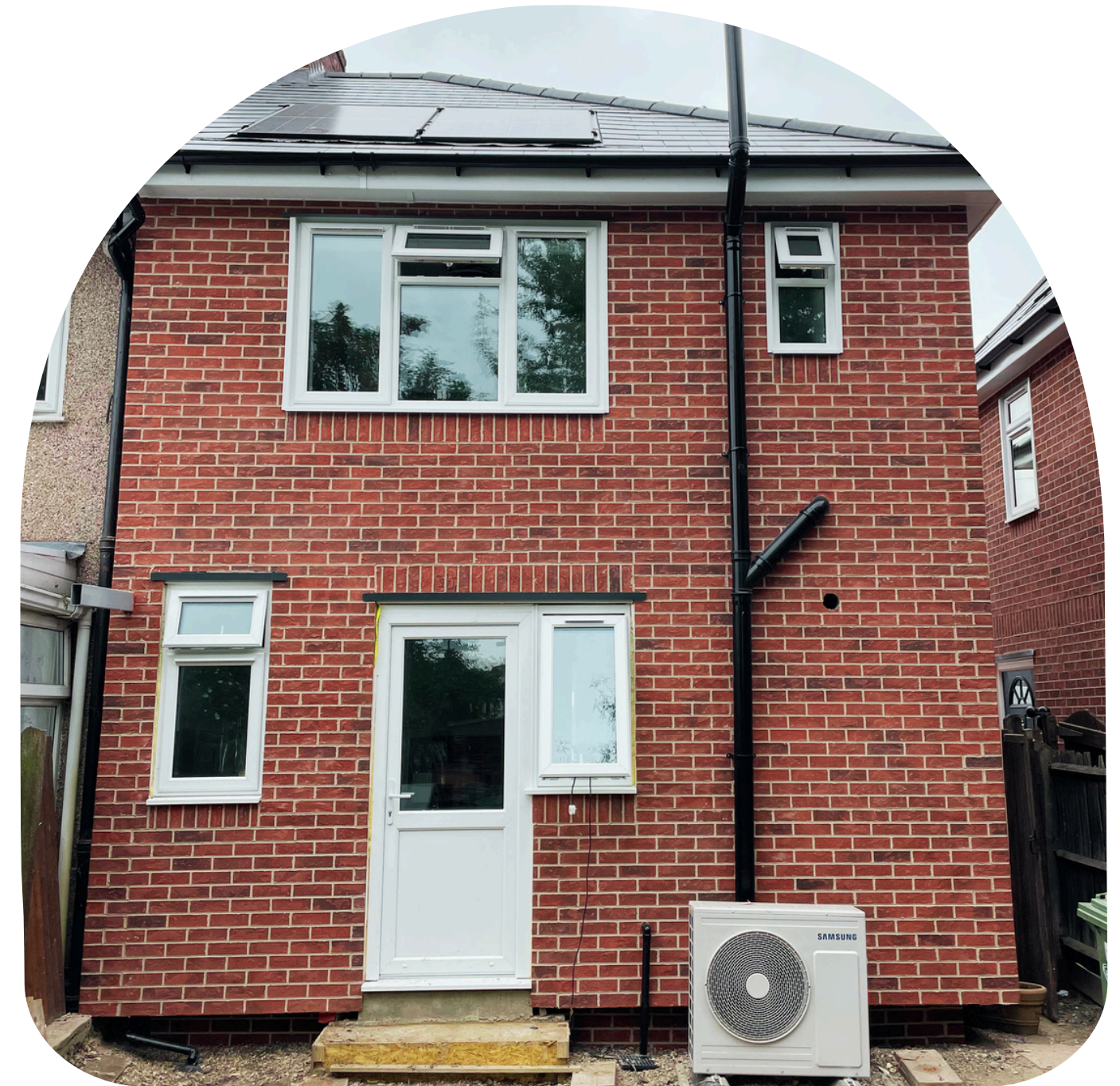
A social home upgraded in the London Borough of Barking & Dagenham. Credit: Energiesprong UK.
