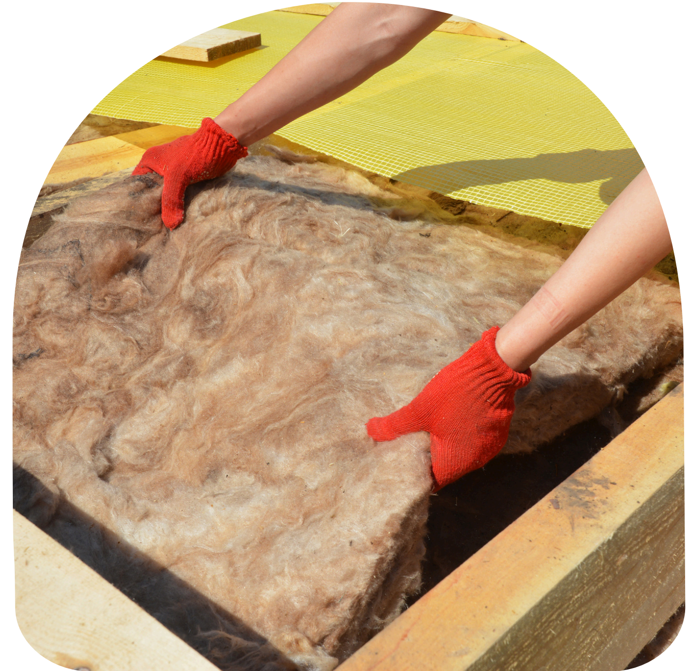
Insulation installation. Credit: Canva stock image
