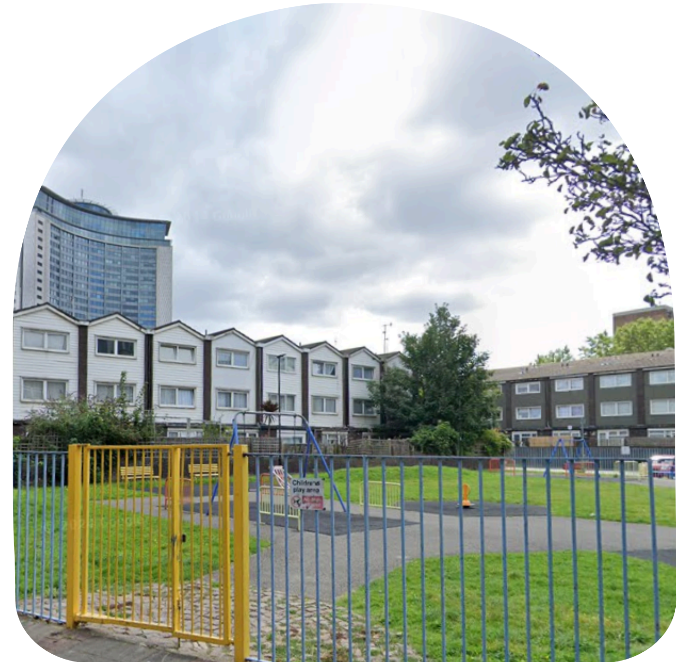
Crosswall homes in the London Borough of Hammersmith & Fulham. Credit: Energiesprong UK
