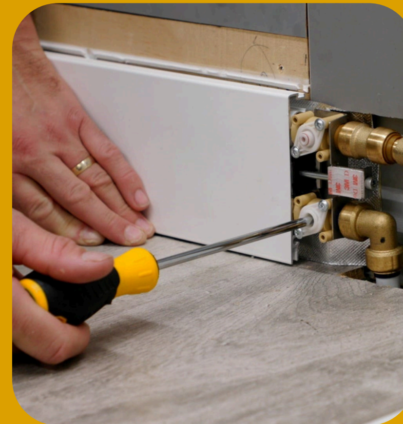
ThermaSkirt installation. Credit: Discrete Heat
