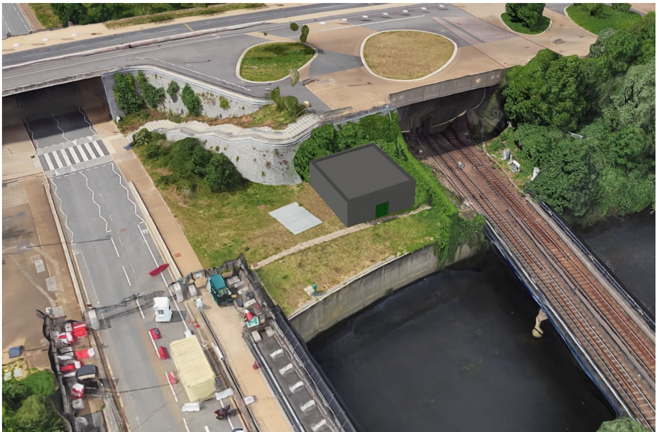
Figure 3-3 – New Pump Room
