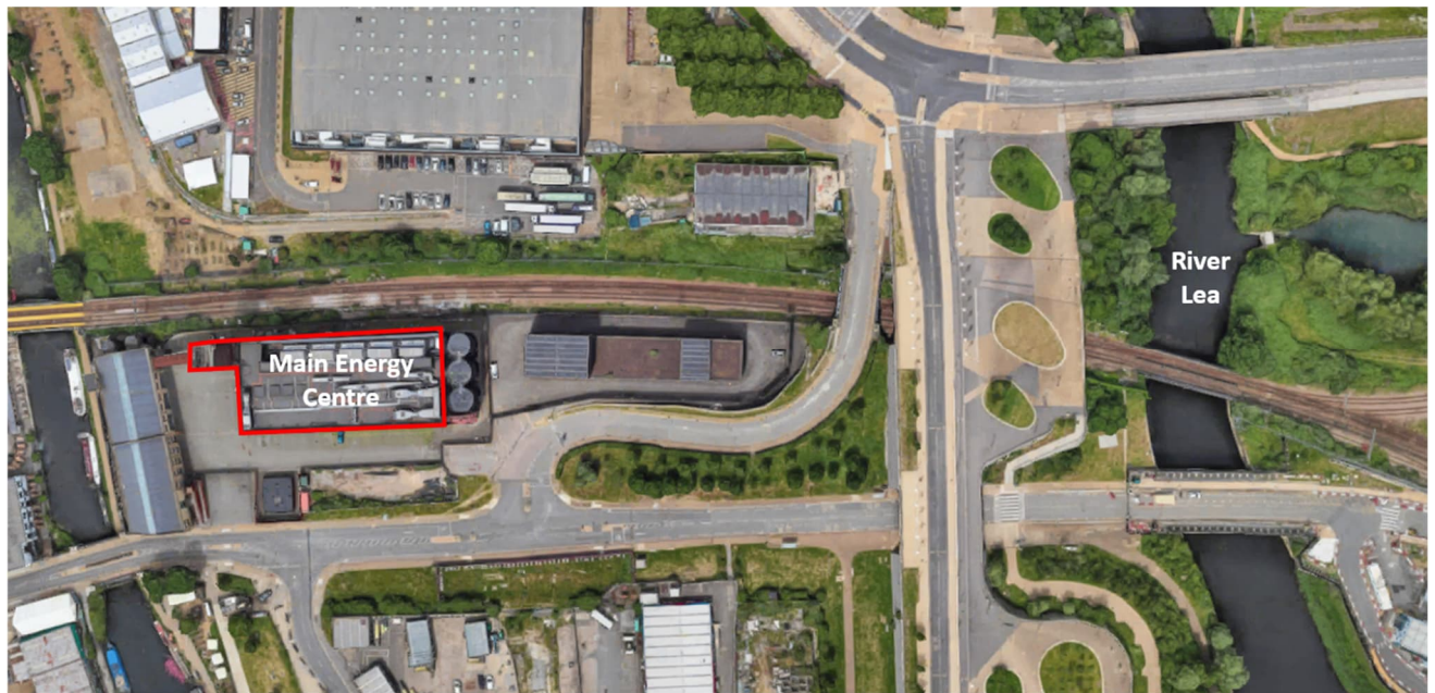
Figure 1-1 - Kings Yard Energy Centre Aerial View
