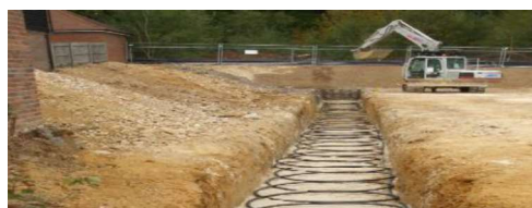
Figure D-12 - Horizontal GSHP arrangement
