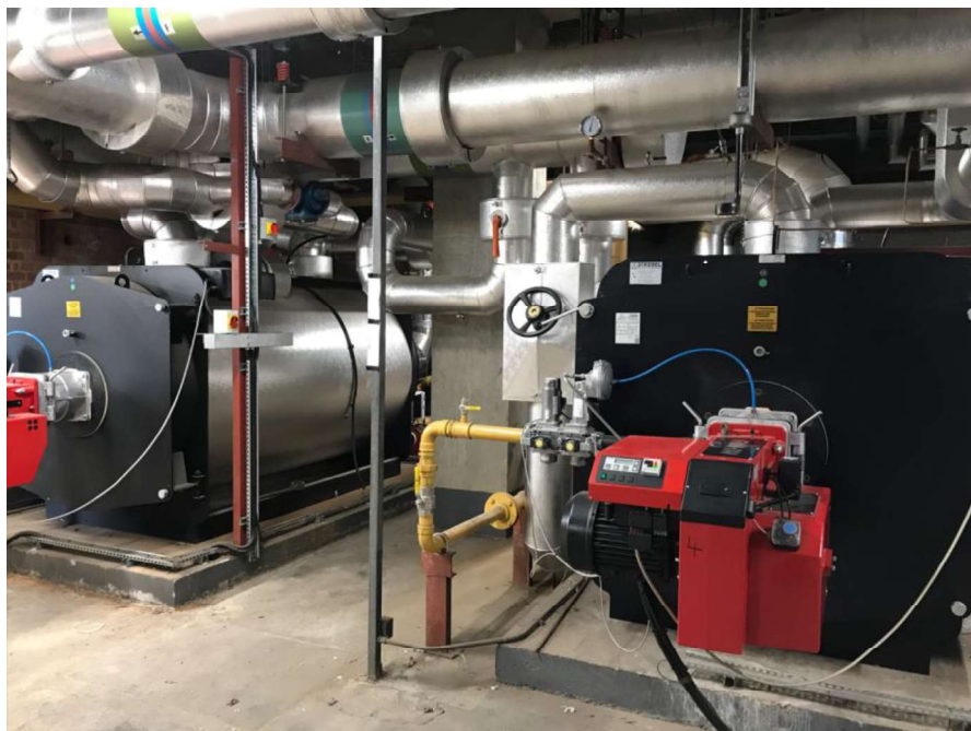
Figure C-2 - Boilers including those that have undergone recent replacement
