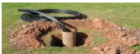
Figure D-13 - Vertical GSHP arrangement
