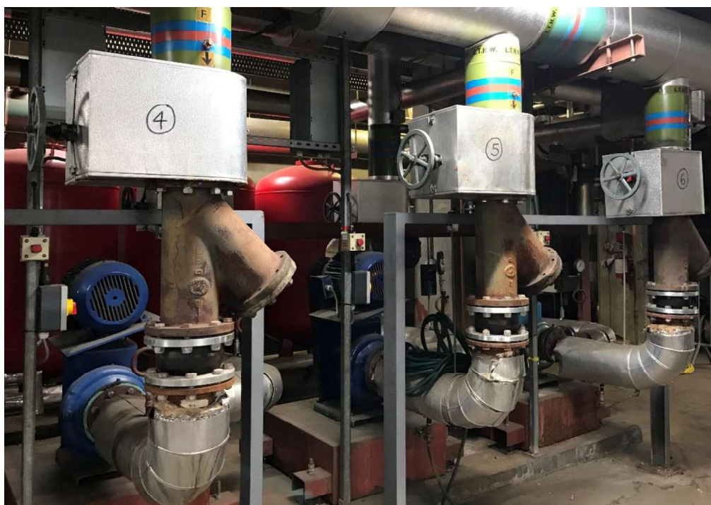
Figure D-8 - Heating circulation pumps in Boiler plantroom
