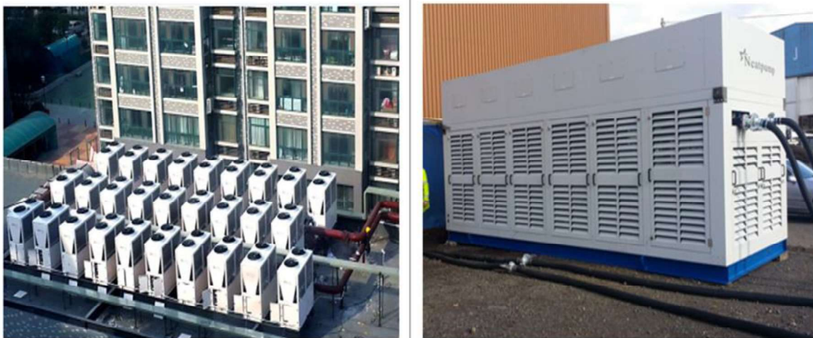
Figure D-14 - Typical ASHP arrangement
