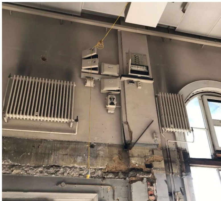
Figure D-7 - Uninsulated pipework
