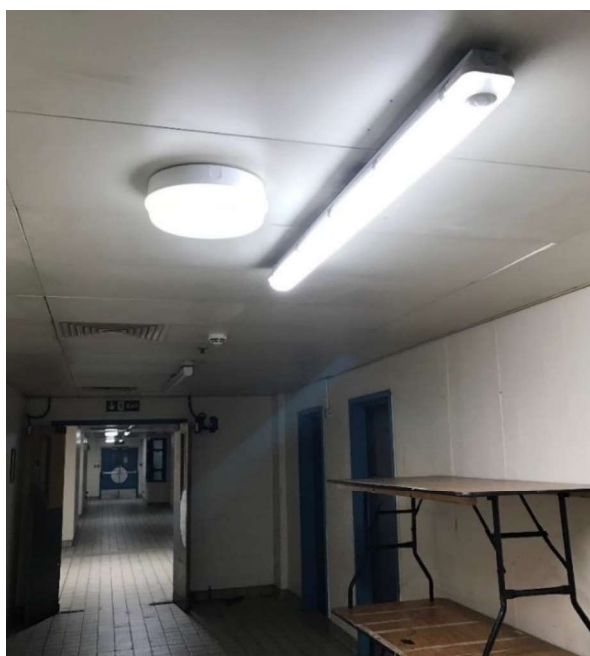
Figure D-2 - Some fluorescent light fittings still await an upgrade to LED
